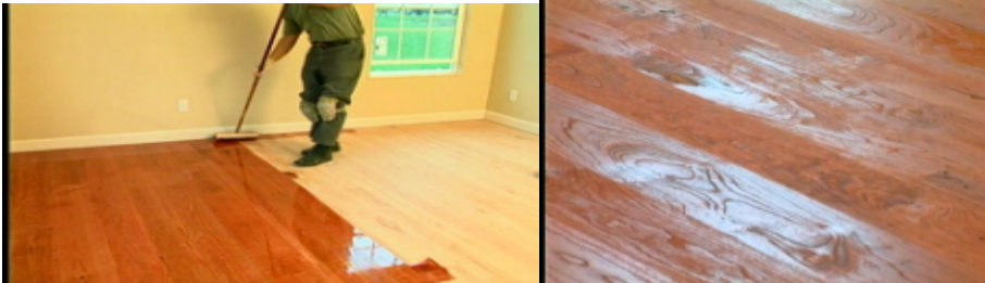
Applying Waterlox Sealer Finish and stain with a lamb's wool applicator
