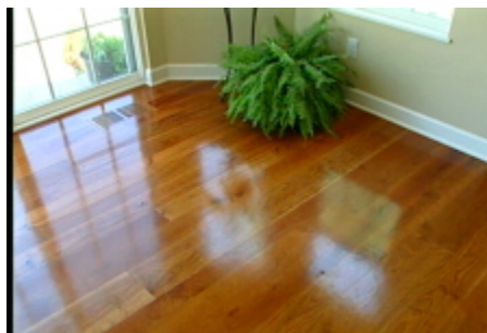
The finished floor with 3 coats of Waterlox Original Sealer/Finish
